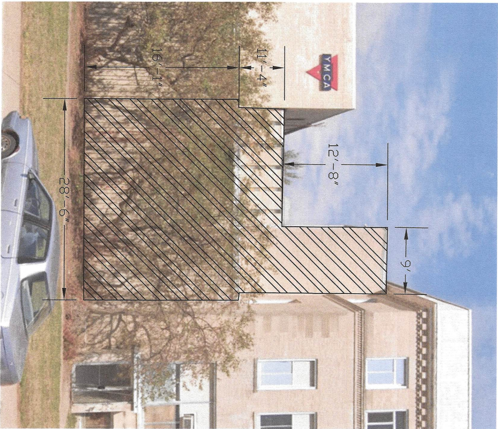
PHOTO OF SECTIONS TO BE REMOVED
