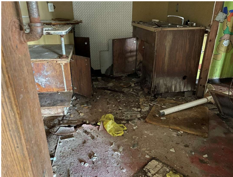
Photo 12: View of Room 6 on the first floor with water damaged materials and delaminated plaster on floor in room
