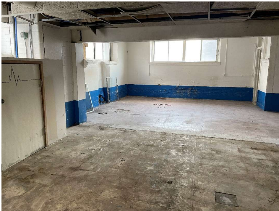
Photo 20: View of significant moisture damage on south wall of basement
