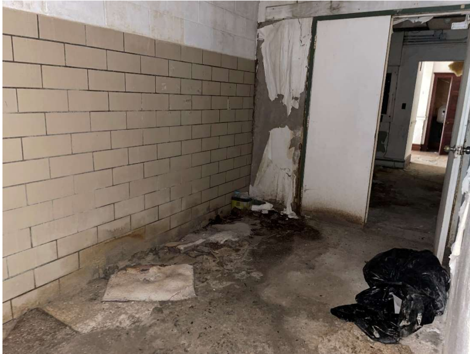
Photo 15: View of second floor north hallway showing significant water damage and staining to various materials
