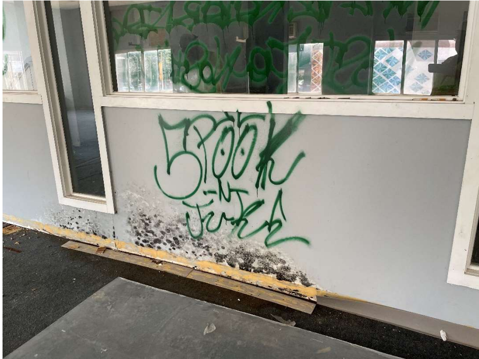
Photo 8: View of observed microbial growth along the north portion of the west wall in Room 4, first floor
