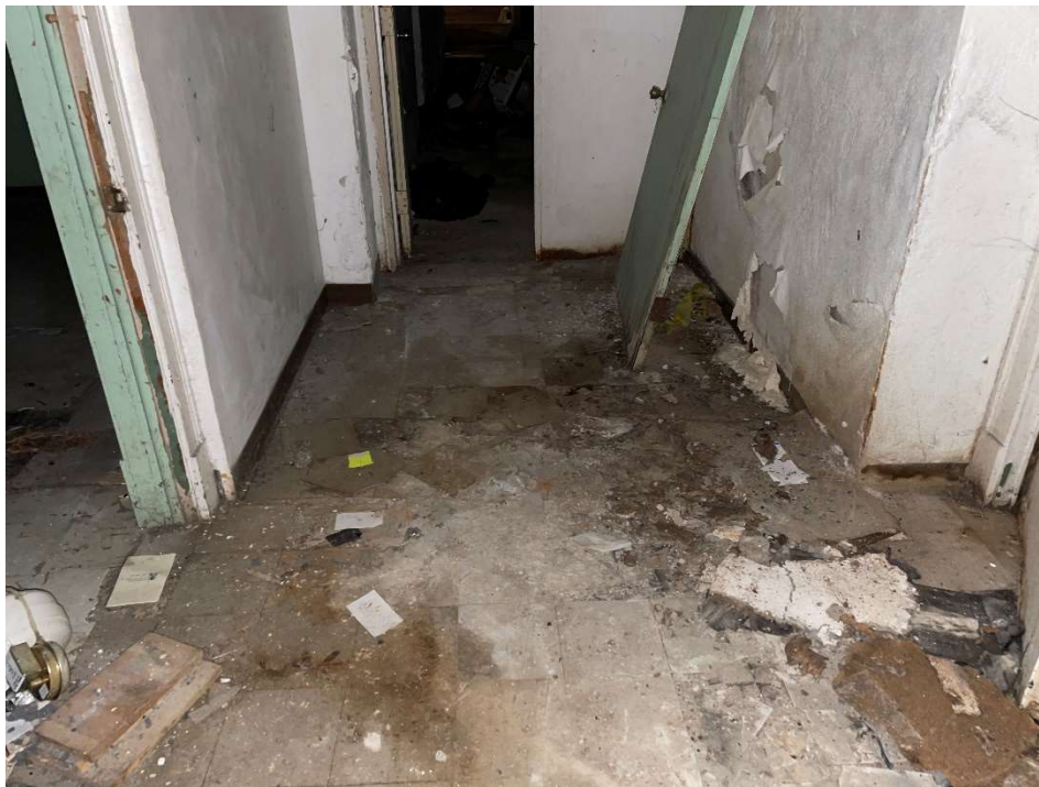
Photo 15: View of second floor north hallway showing significant water damage and staining to various materials
