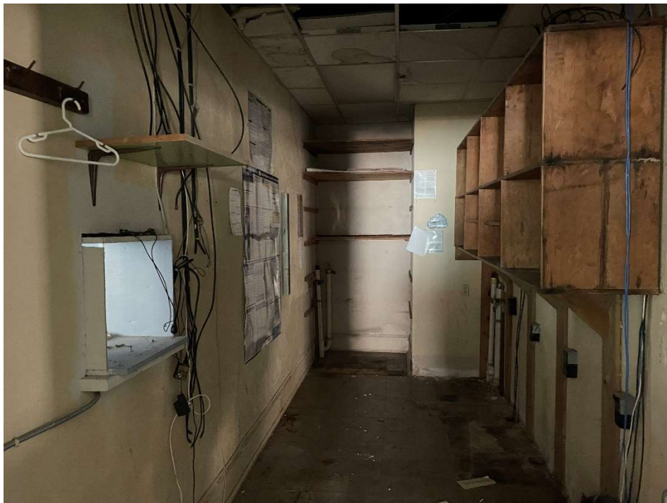
Photo 10: View of Room 3 on first floor with water stained ceiling and floor tiles
