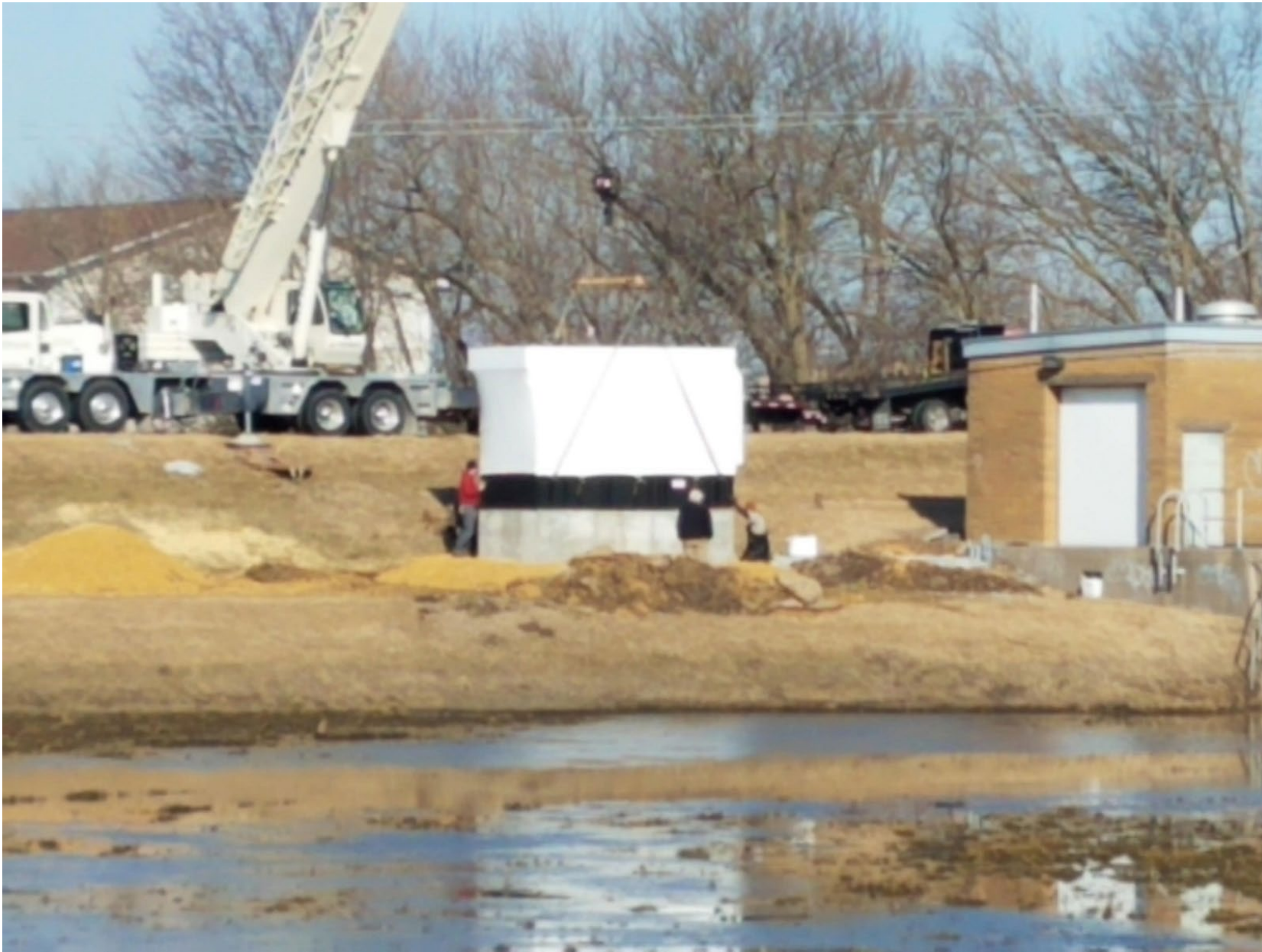
Setting the stand by generator at the Millcreek flood station
