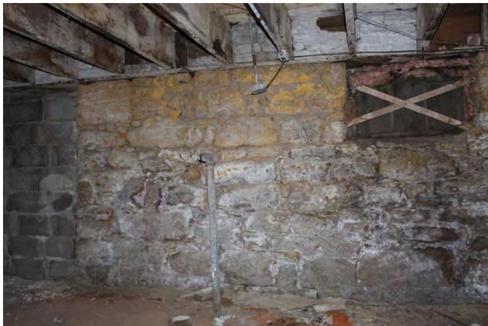
Property Photograph 10 – Potential UST pipe in basement of 1000 S. 4 th St.
