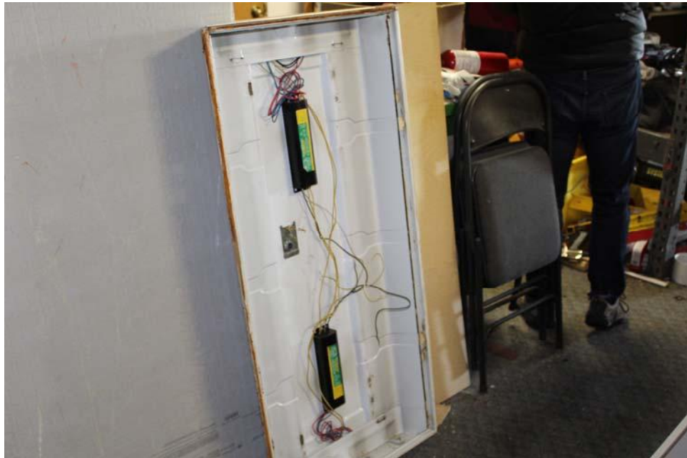
Property Photograph 19 – Fluorescent light ballast on 1 st Floor at 1004 S. 4 th St.
