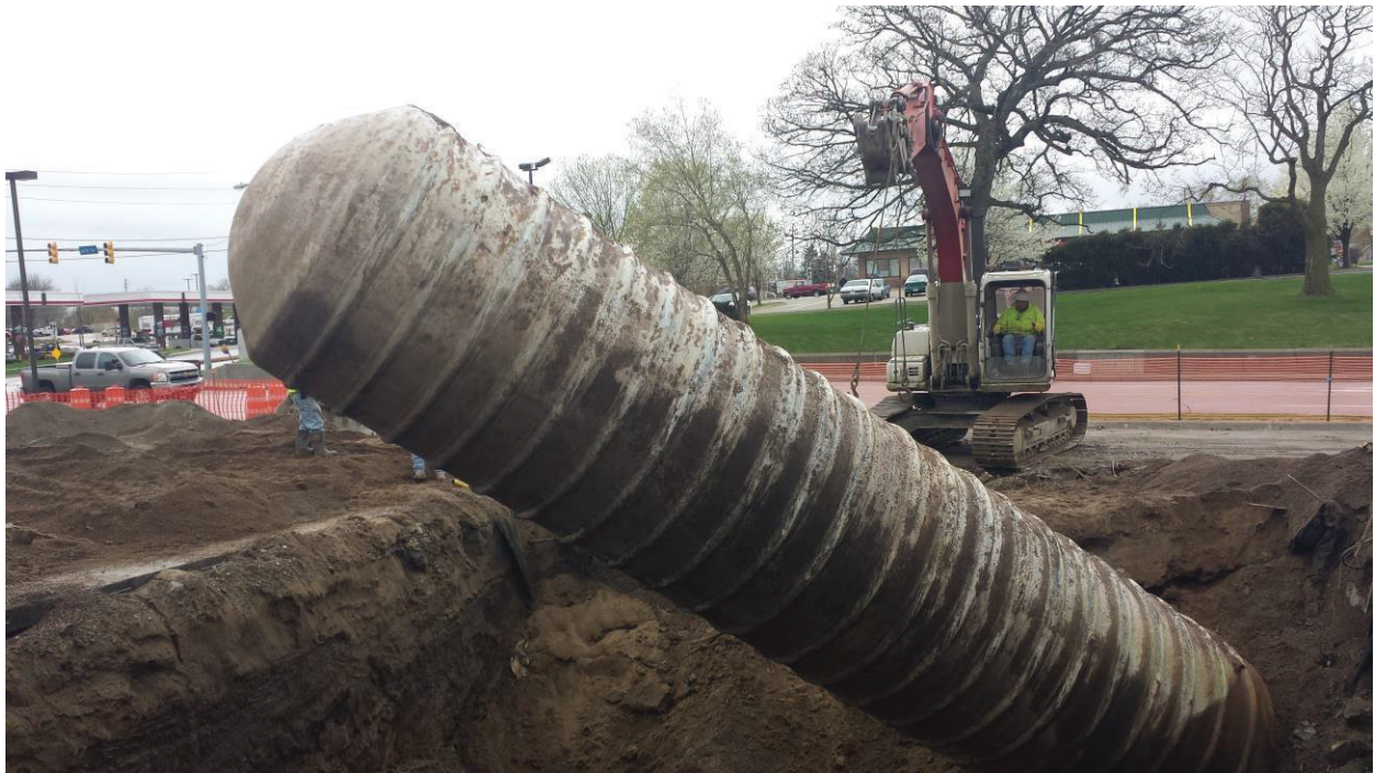
12000 gallon double wall Xerxes fiberglass tank removed in May 2014 at QuikTrip, 6 th and University Avenue, Des Moines.
