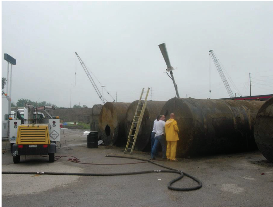
Photo of eductor in operation at a Des Moines tank removal. Purging should continue as long as possible to keep vapors from regenerating in the tank.
