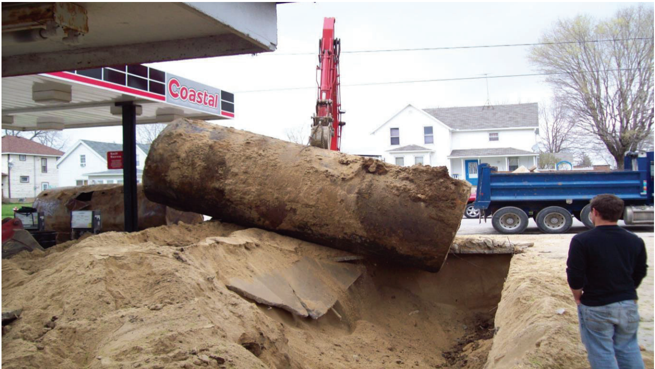
Tank removal in Waukon. Planning a tank removal must take into account overhead power lines and canopies that can present risks for removers. Please note, the person standing close to the excavation is not wearing safety equipment and the excavation is not barricaded.
